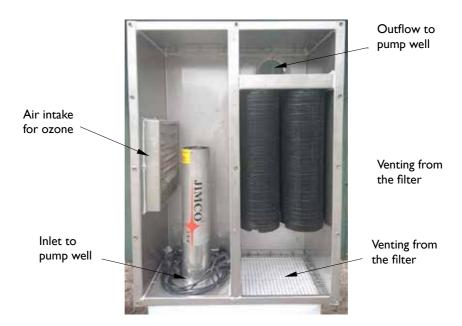
In the hydrogen sulfide filter over ground, the HS Purifier is placed so the UV-C produced ozone gets access to the pump well and is supplied to the well using the HS Purifier's ventilator.
